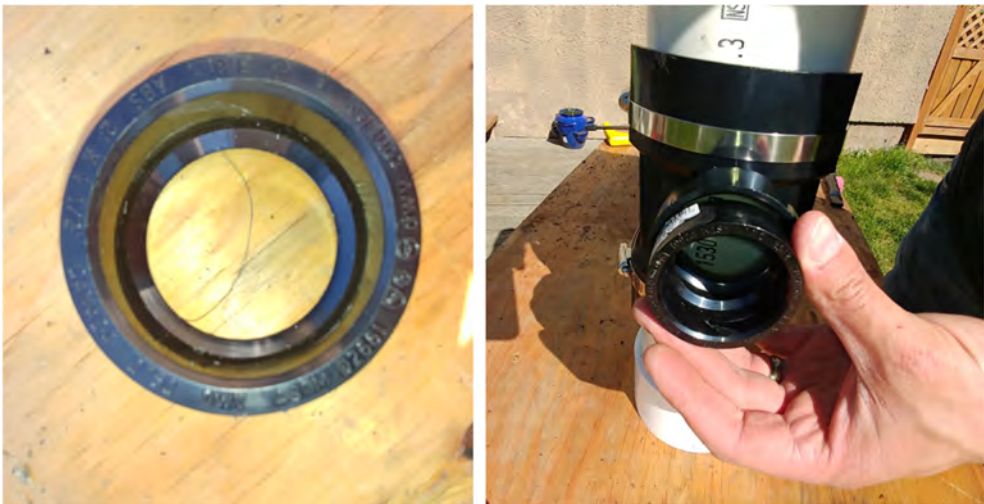
Fig. 32. Installation of the bushing on the tee fitting.
