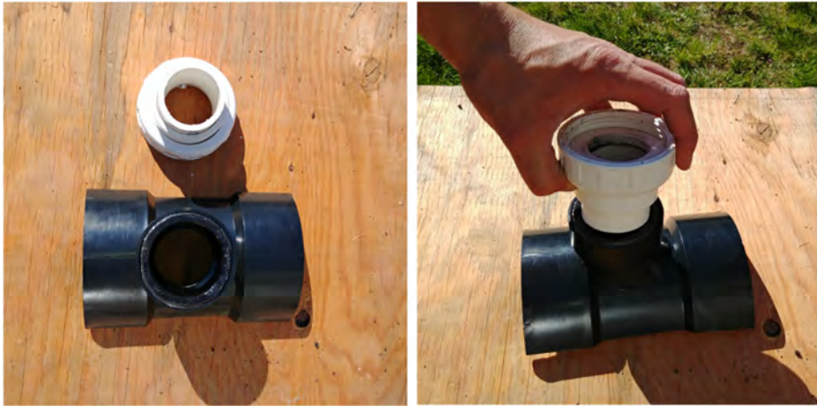
Fig. 33. Installation of the PVC union fittings.
