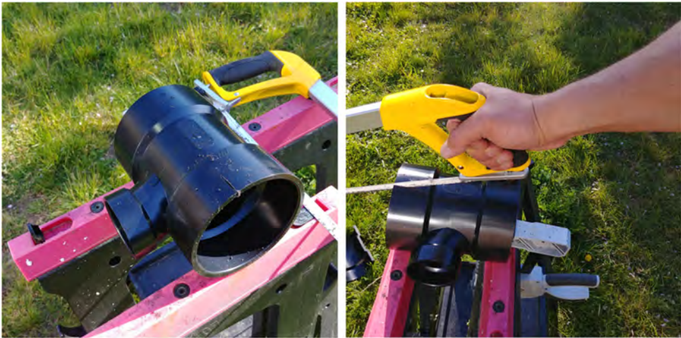
Fig. 31. Cutting of the tee fitting.
